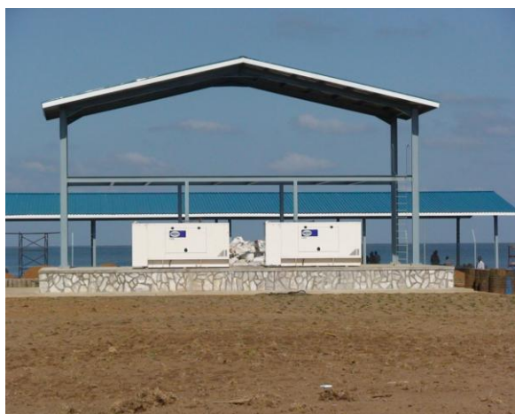
Constructed shade at Mweena in Kalangala
