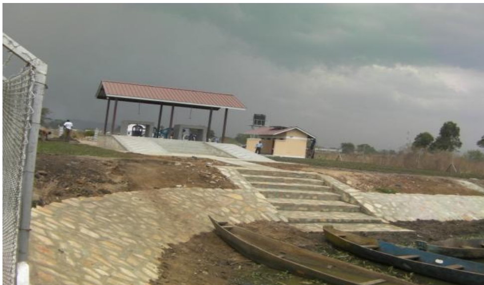
Figure 7.2: Ntoroko Landing under Construction
